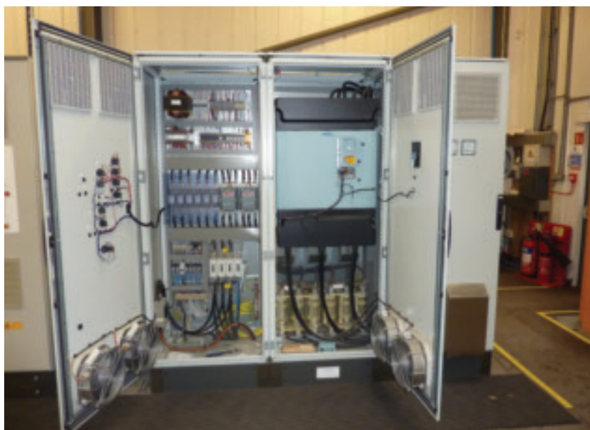
Figure 1. The Vacon software allows drives to store multiple parameter sets, with the parameter set required in any particular instance selectable via the drive's digital inputs.
