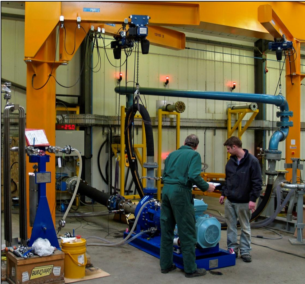
New Amarith test facilities
