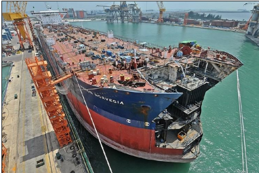
Conversion of the Navion Norvegia into Pioneiro de Libra FPSO at the Jurong Shipyard of Singapore
