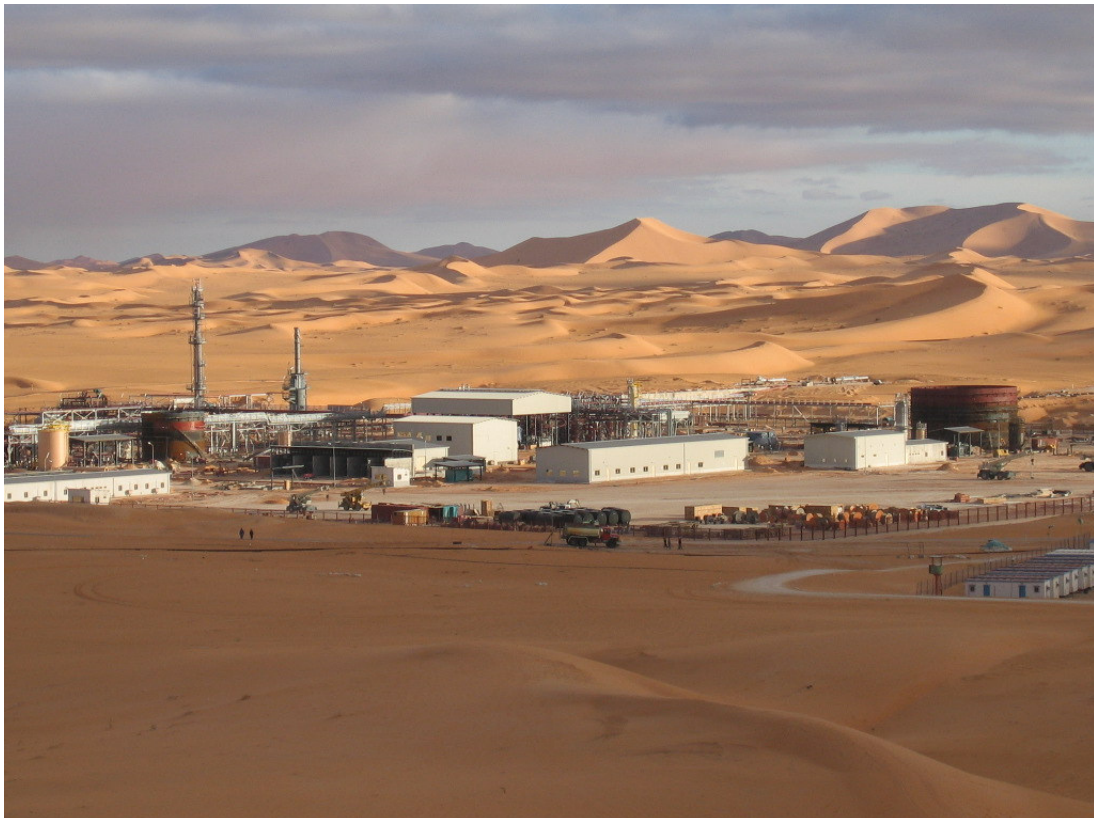
The Sonatrac site at Birbirkine, Algeria
