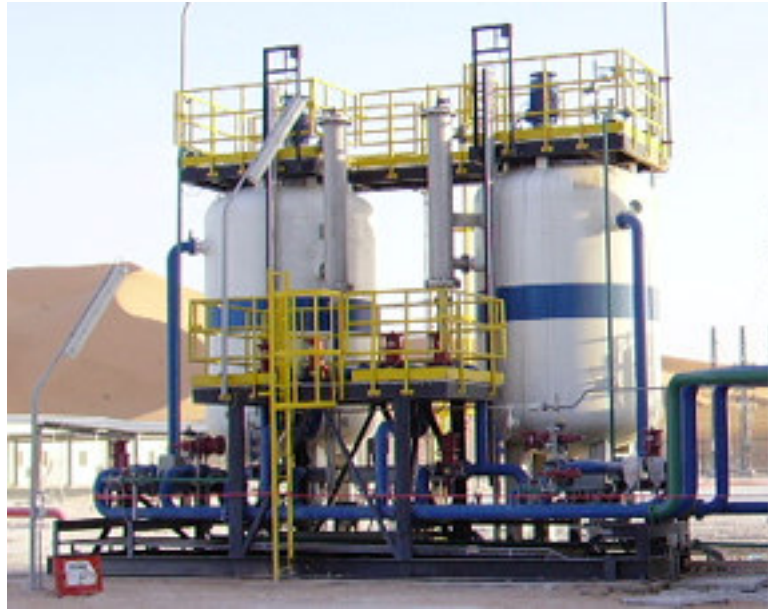
Axsia nutshell filters in-situ
