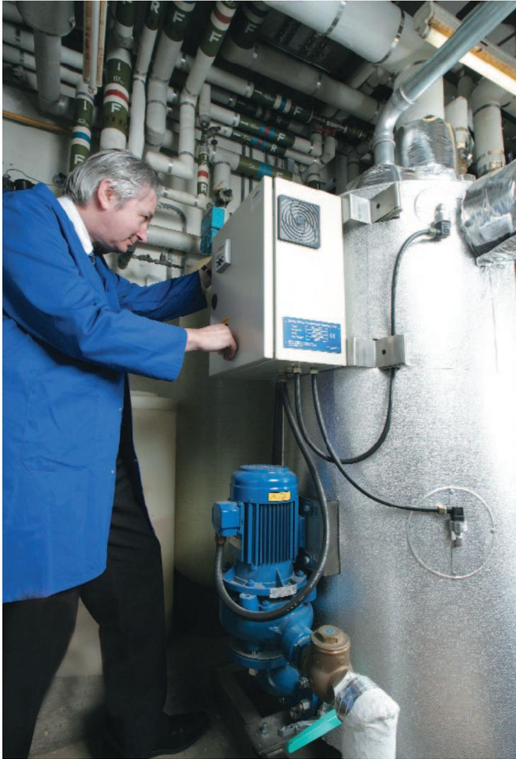
**An effective condensate recovery system will collect hot condensate from the steam system and return it back to the boiler plant to be used as boiler feed.**
